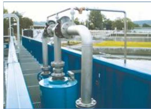
Swivel joints will be used when you have to convey fluids from a fixed point to parts in relative motion and meets virtually all industrial applications.
